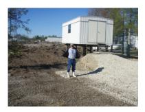
Figure 19: Storage Shed #1 was raised 6 ft on pilings and provided ramp access (\$3,700) (Oct 2008).
